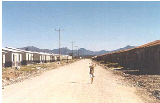
Fig. 5. View of a suburb-like resettlement in Nueva Choluteca, where no roads, sidewalks, or infrastructure were completed.
