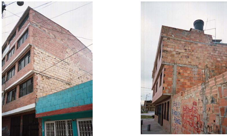
Fig. 3. Successive cantilevers and multiple floors are built in the construction process, sometimes (like in these pictures) without the use of concrete columns.
